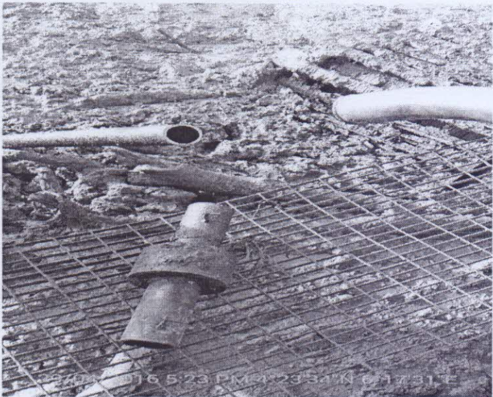
POINT DURING REPAIR SHOWN: fig2
